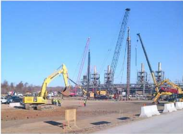
Ground breaking at Clear Lake, Texas methanol site in foreground
